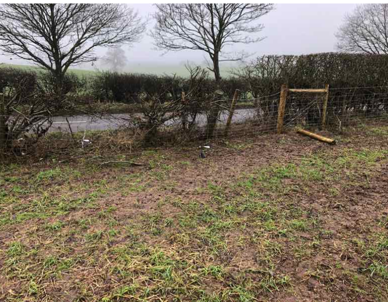
Figure 19: Evidence of field boundary damage (continuous along the identified road stretch) leading to livestock escaping into road.
