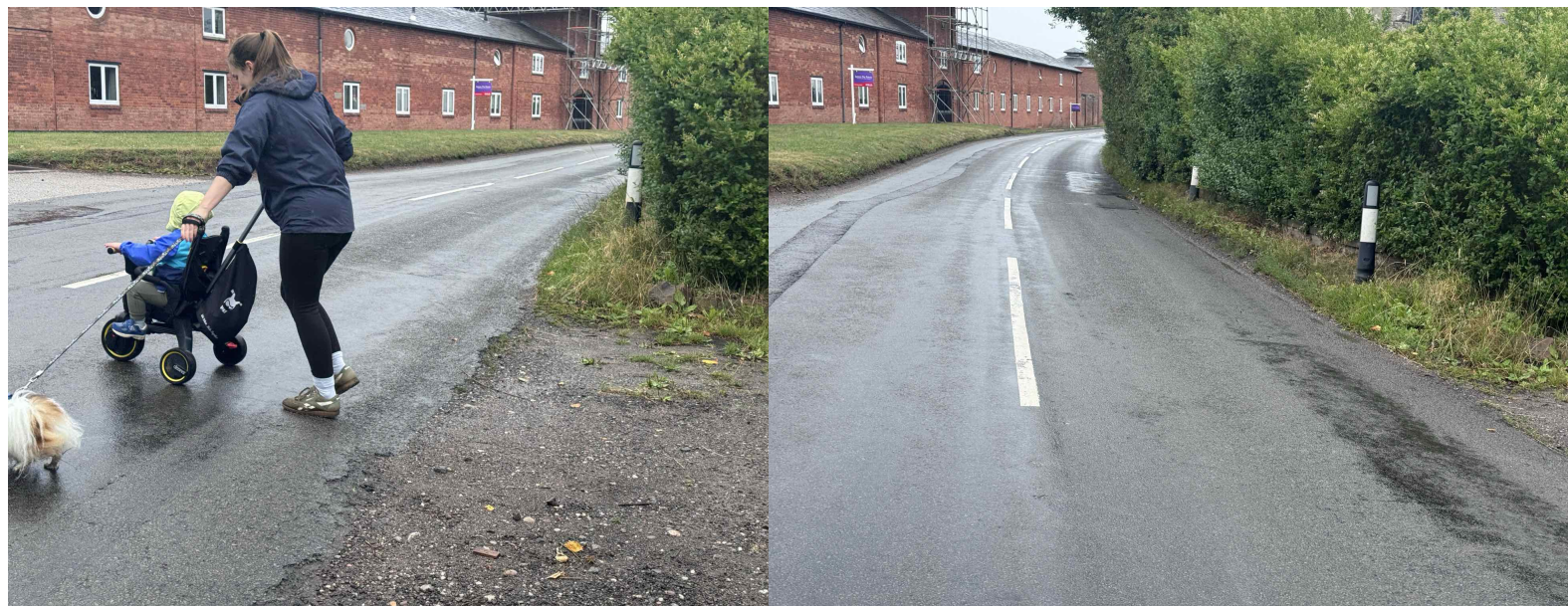
Fig. 6 a/b As pedestrians and horse riders commit to crossing, the approach from oncoming traffic is still blind due to road curvature. (B) Still no clear view of fast traffic in the centre of the road.
