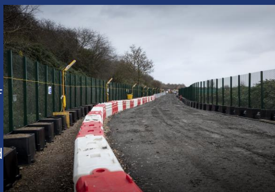
A haul road constructed for Phase One of HS2
